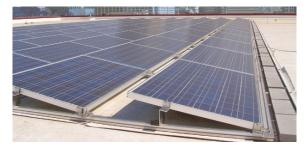
Fig. 3.3.4: Ballasted footing mount structure
